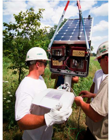
The Carmanah EverGEN 1710 units are compact, self-contained and designed to install in 30 minutes or less.
