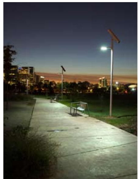
Carmanah solar LED lighting provides a compact, self-contained design that blends easily into aesthetic environments such as Juan Pablo II Park.
